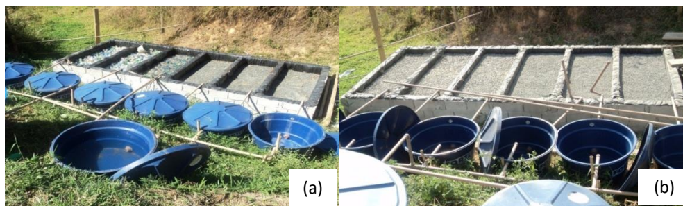
FIGURE 3. Overview of the six HSSF-CWs, three filled with PET bottles; and three filled with gravel # 0 (a) and after placement of the cover layer with gneissic gravel # 3 (b).
