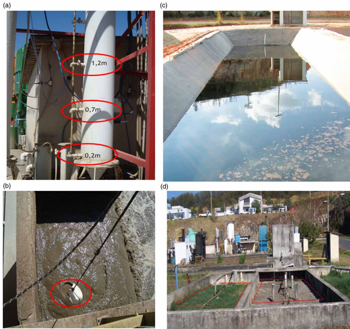
Figure 1 | Sewage treatment systems investigated: (a) pilot-scale UASB reactor; (b) activated sludge system (return sludge); (c) polishing pond; (d) vertical flow constructed wetlands.
