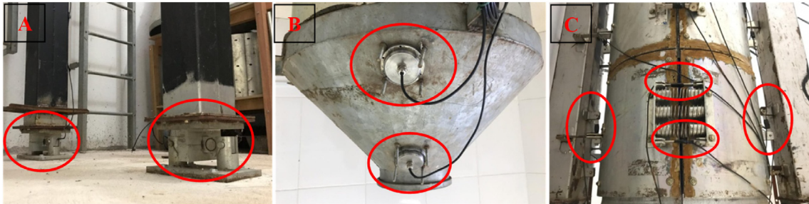
Fig. 6 – Location of measurement cells in the pilot silo. (a) Shear beam load cell, pillar base; (b) pressure cell, bottoms; (c) tension load cell, silo rings (vertical - friction, horizontal - normal).
