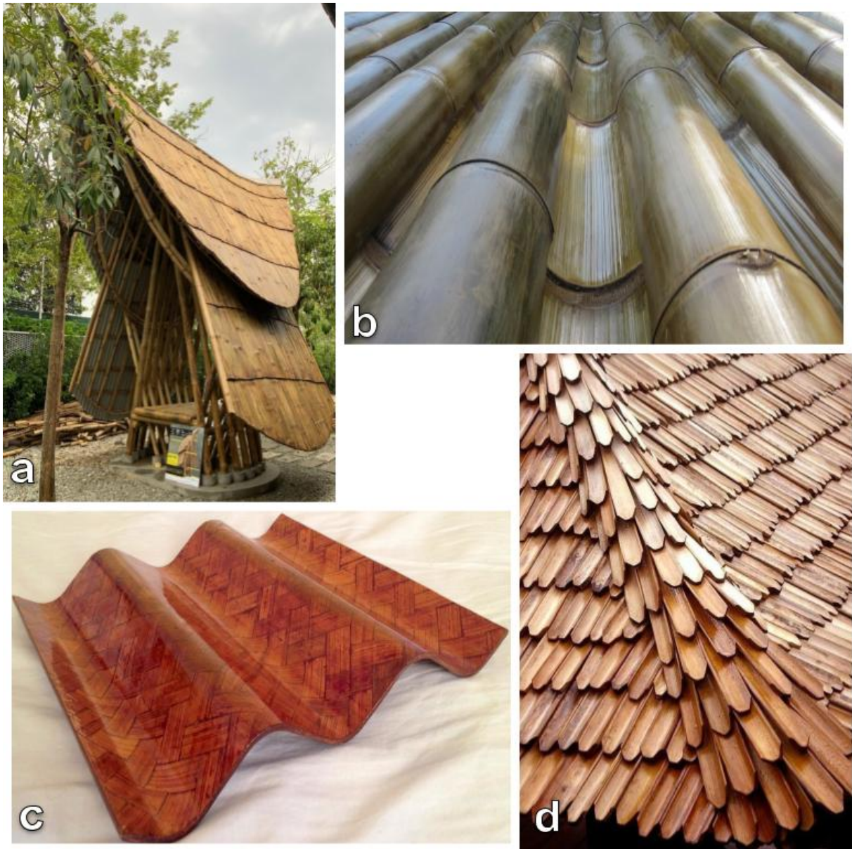
Figure 28 – (a) three-layer bamboo roof shingles. (b) Bamboo culm half-pitched roof. (c) Corrugated bamboo roofing sheets. (d) Slatted scale roof.
