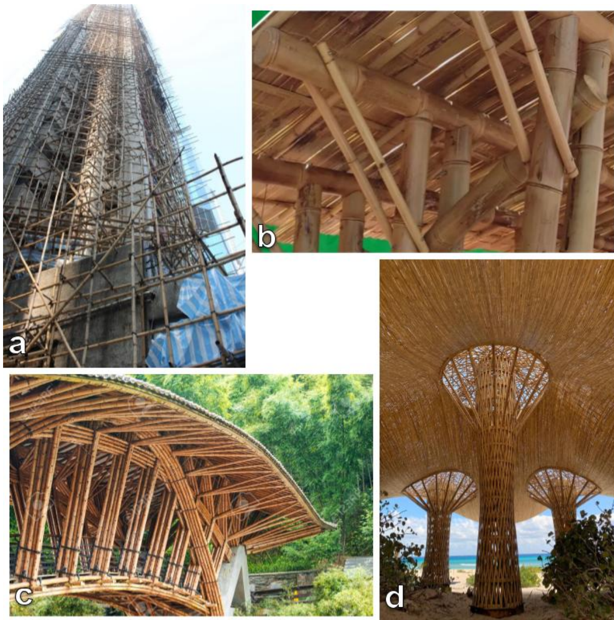
Figure 26 - Bamboo in various construction uses such as: (a) scaffolding, (b) structural trusses, (c) covered bridges, and (d) complex three-dimensional bundle structures.
